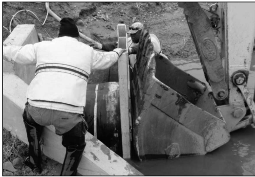
Pallet Push method for installing CheckMate® Valve
